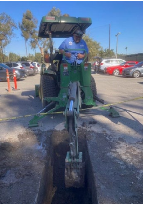
CREWS WORK TO REPAIR A WATER LINE BREAK AT THE RECREATION DOG PARK
