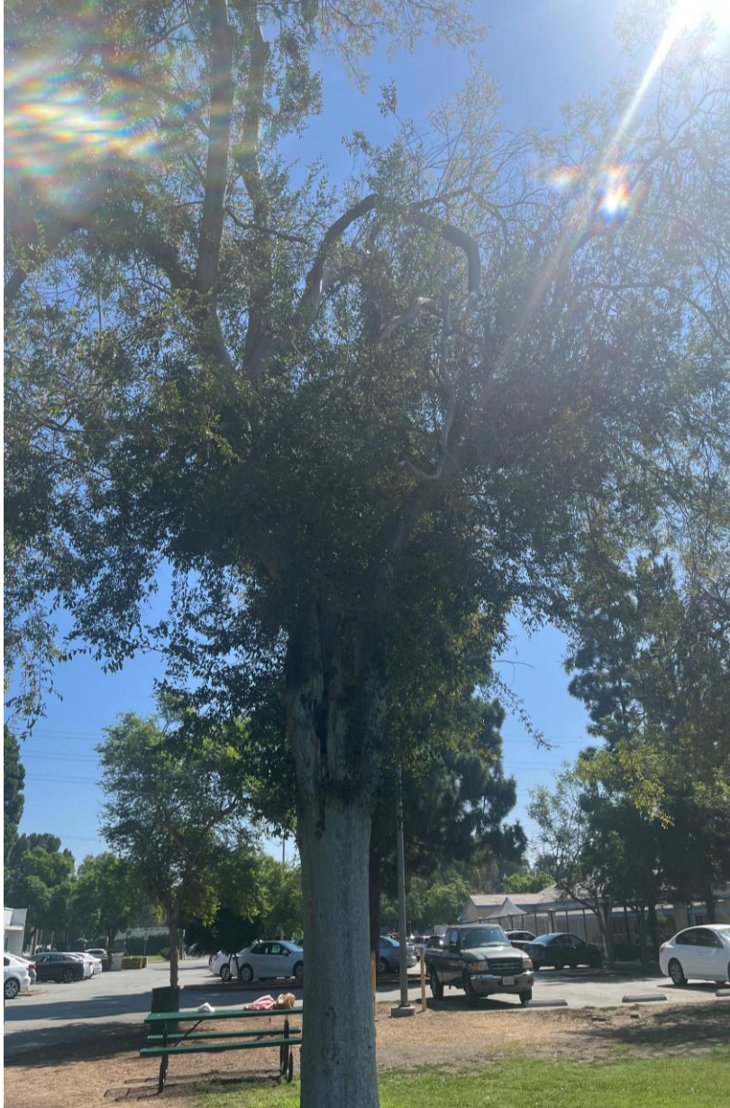
Tree in overall decline. Tree has a severe cavity on the primary leader. Making structurally unsound. Base of the tree beginning to decay.
