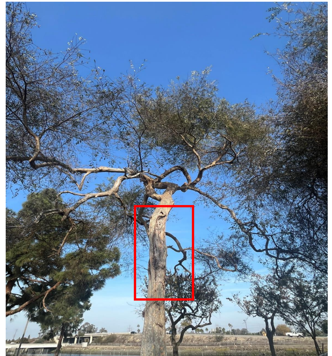
The tree was trimmed to prevent removal. Work was unsuccessful due to broken limb and poor tree structure. Trunk shows advanced stages of anthracnose.
