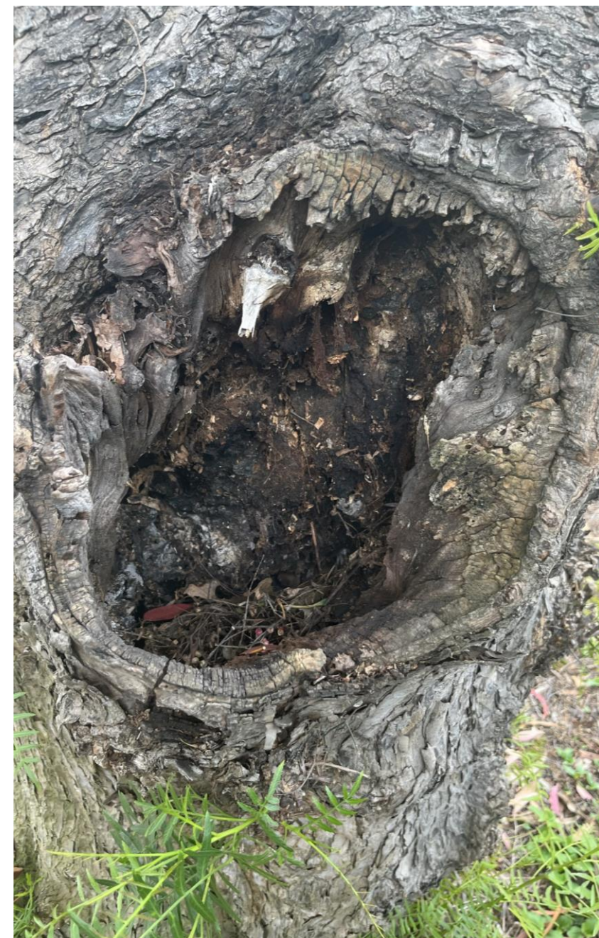
Close up of the cavity
