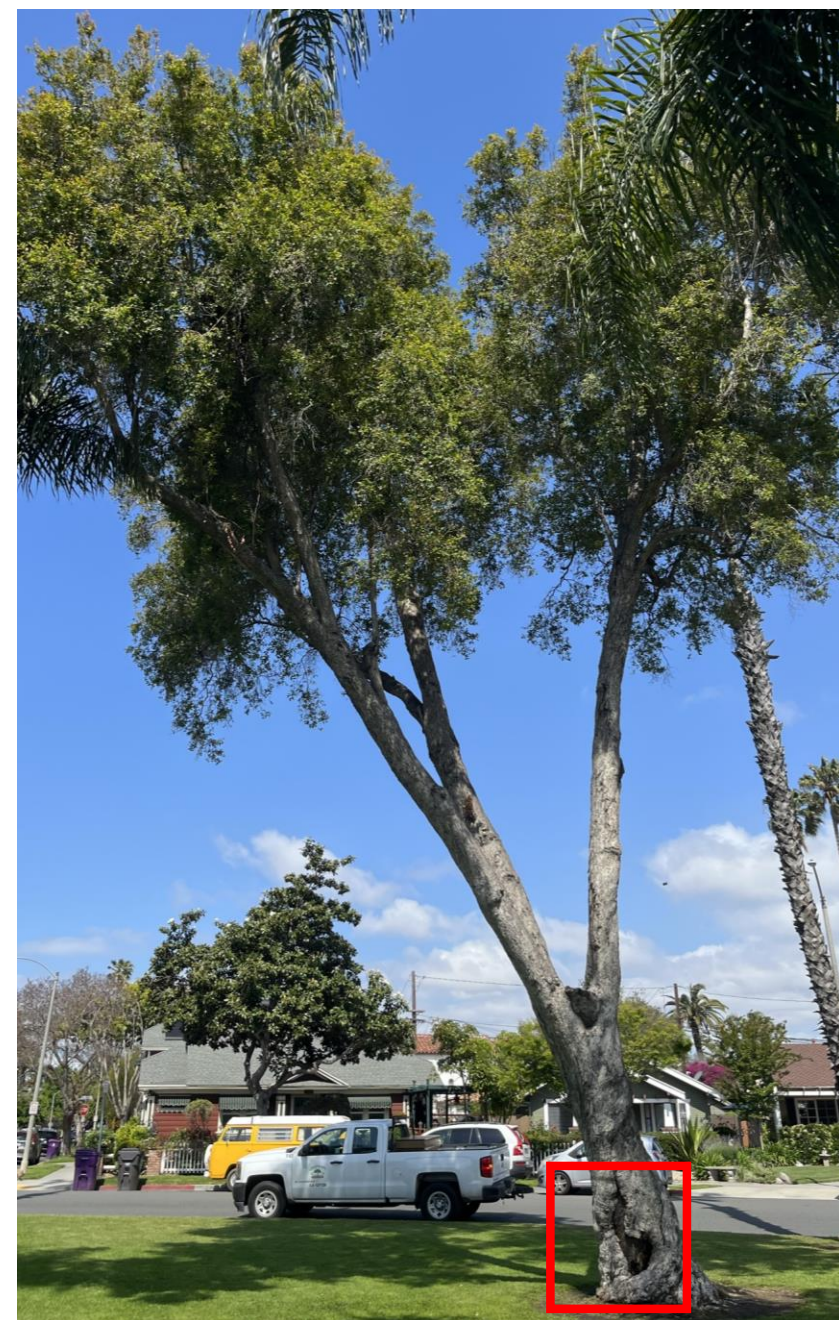
Overall photo of the tree with the cavity in the main trunk.
