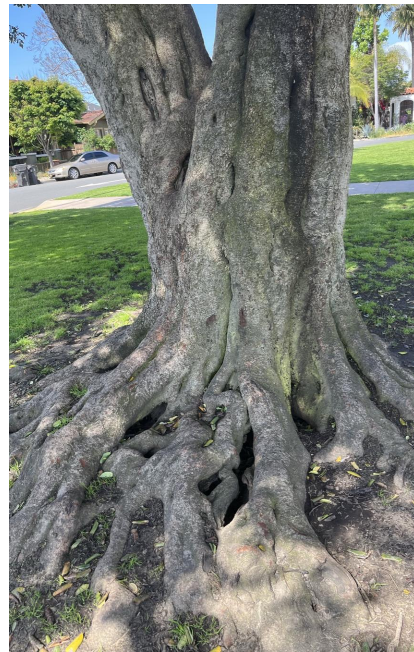
Roots beginning to lift.
