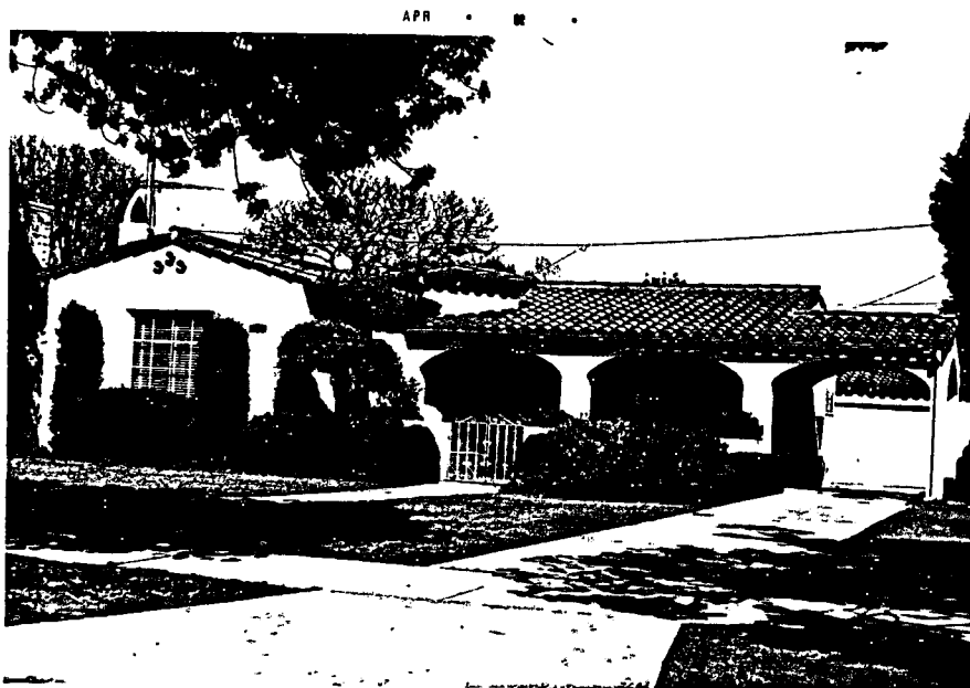
4230 LINDEN AVENUE (1938) - Spanish Colonial Revival stucco cottage with a low pitch intersecting gable tile roof. Segmental arched forming driveway and front patio. Square low tower with pyramidal roof. Contractor, L. H. Mussetter. (Photo BK2-16)
