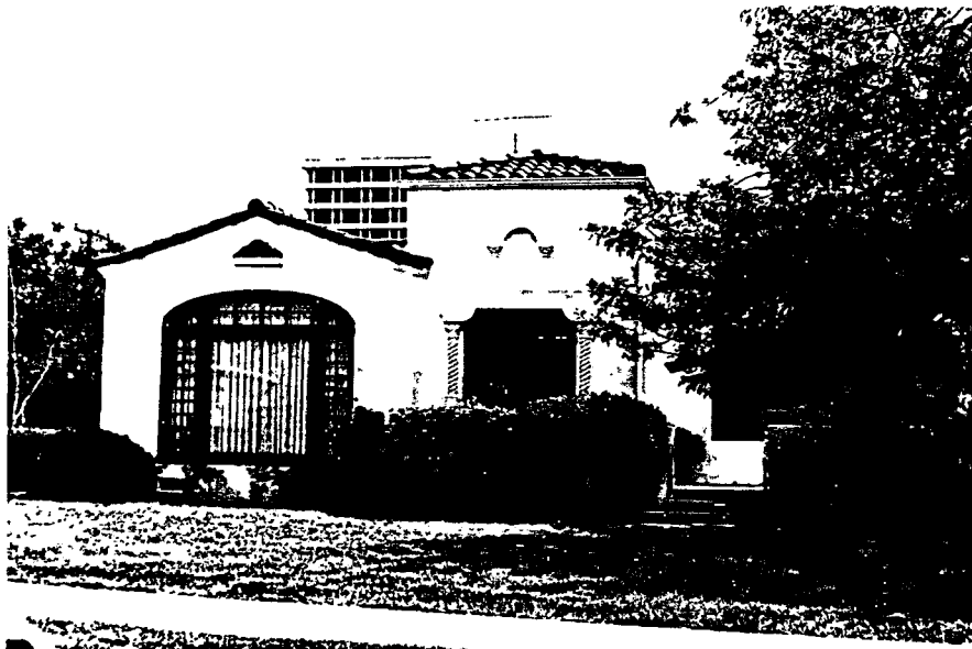
3720 ELM AVENUE (1925) - Spanish Colonial Revival stucco cottage with a low pitch intersecting gable tile roof and large square entry tower with pyramidal roof in front. Large segmented window with multi-paned transom and sidepanels. Spiral molding on the sides and top of structural opening. Contractor, Hinte & Son. (Photo BKL-5)
