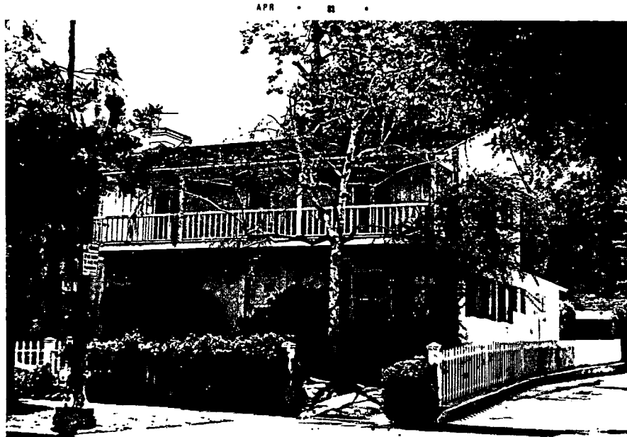
4301 LINDEN AVENUE (1931) - Monterey Revival style two story structure with wood shingle gable roof. Stucco on lower level and board and batten on upper level. Shutters on multi-paned windows, double screen doors on entry to second story balcony with wood rails, and shelf pediment over main entry. Contractor, Wm Tosh. (Photo BK2-18)
