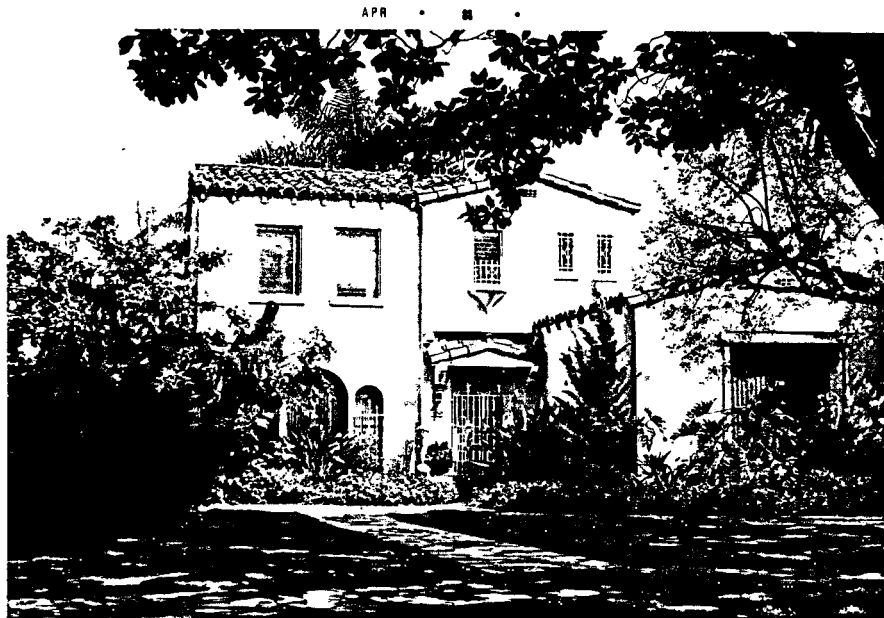
4200 LINDEN AVENUE (1935) - Spanish Colonial Revival two story cottage with a tile gable roof. Front gable extension with large square window framed with turned wood and plain lintel. Tile gable pediment with brackets over entrance. Owner/Contractor, Adelaide Bowman. (Photo BK2-13)
