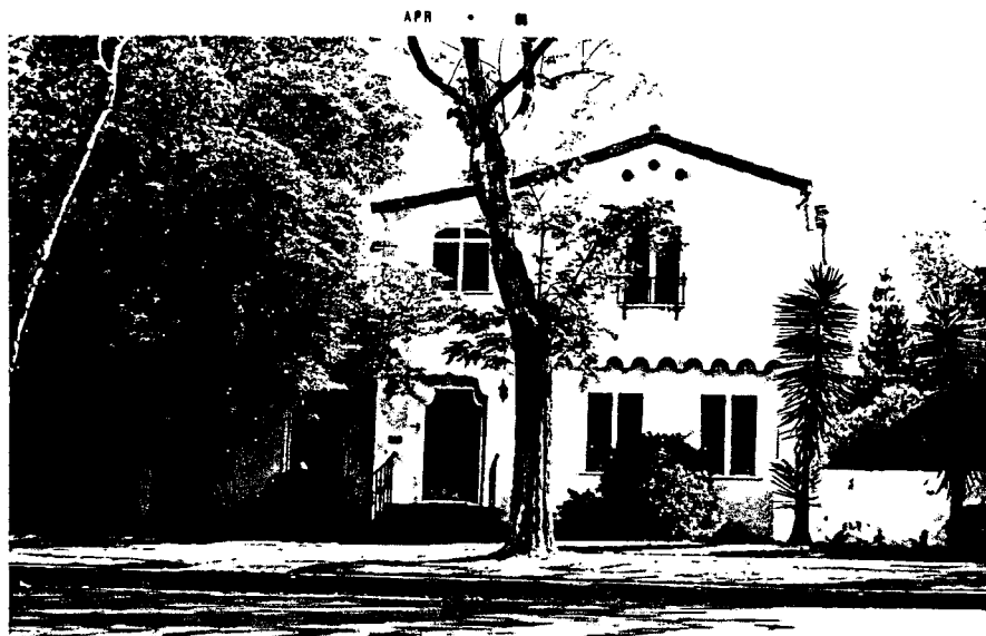
4019 LINDEN AVENUE (1929) - Spanish Colonial Revival two story stucco cottage with a tile gable roof. Mission style recessed structural opening at entry. Series of small arches segmenting the first and second story. Two sash vertical windows. Owner/Contractor, B. L. Thurber. (Photo BK2-5)
