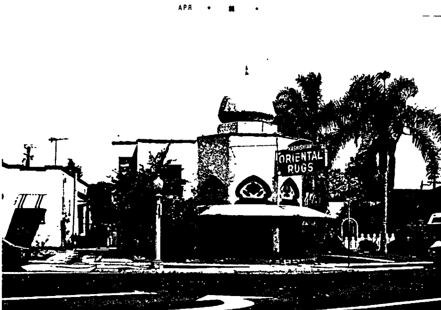
401 E. CARSON STREET (1937) - Hollywood Islamic stucco 2 story commercial structure with a flat roof capped in tile. Octagonal front portion extending the full 2 stories with 4-center ogee decorated cut-outs on each facet. Large conical ornament with finial on top of building. Design theme extended on side yard fence. (Photo BK1-19 & BK3-10)
