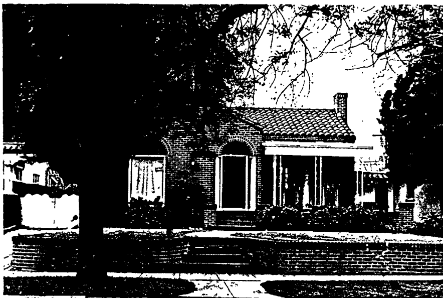
3817 LINDEN AVENUE (1929) - Spanish Colonial Revival brick cottage. Arched front window with blind single fanlight. Glass single fanlight over entry. Two double sash french windows with spoked fanlights under aluminum awning. Contractor, Sid J. Spearin. (Photo BKL-25)
