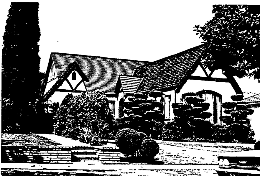
3905 LINDEN AVENUE (1930) - Period Revival stucco cottage with a wood shingle intersecting gable rolled edge roof and imitation half-timbering. Gable dormer-type entry with radiating brick arch. Segmented vertically divided front window. Noteworthy landscaping. Contractor, A. E. Forman. (Photo BKL-32)
