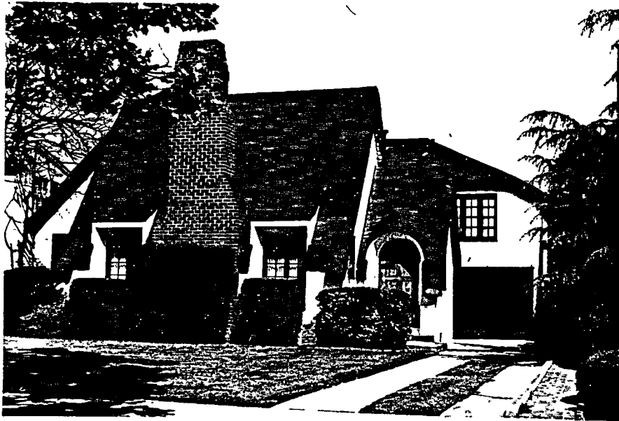
4126 LINDEN AVENUE (1932) - Hansel and Gretel stucco cottage with a high pitch rolled edge composition shingle roof. Gable entry extension with an arched recessed entry forming a swept roof line. Shed dormer-like recessed multi-paned double sash window in front and carriage type garage doors with transom windows. Large irregular shaped chimney. (Photo BK2-9)
