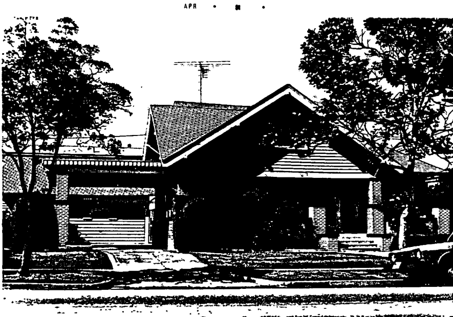
323 E. BIXBY ROAD (Circa 1910) - California Bungalow with medium pitch composition intersecting gable roof and horizontal wood siding. Multi-sash and transom windows on lower story and diamond patterned window in upper gable. Brick porch and carport supports. Garage door window. Contractor, Earl L. Chessman. (Photo BK2-19)
