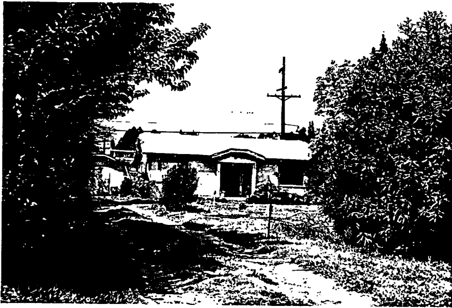
3945 ELM AVENUE (1923) - California Bungalow with a clipped gable composition roof and large one sash windows. One car garage roof to match front porch cover. One story. (Photo BK1-12)
