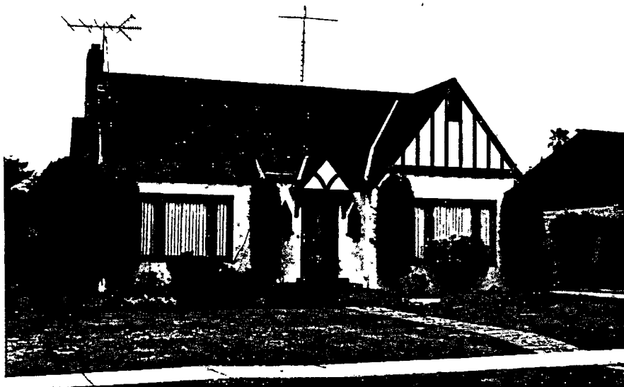
3719 LINDEN AVENUE (1925) - Period Revival stucco one story cottage with a high pitch wood shingle gable roof and imitation half-timber in the front gable. Gable pediment (also half-timbered) with brackets over entry. Three sash windows with upright dividing bars. (Photo BKL-21)
