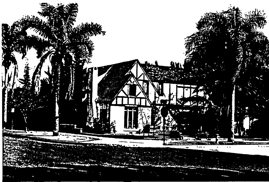
4020 LINDEN AVENUE (1929) - Period Revival stucco 1 1/2 story cottage with imitation half-timbering and a high pitch wood shingle intersecting gable roof. Multi-paned windows. Recessed arched entry. (Photo BK 2-6)
