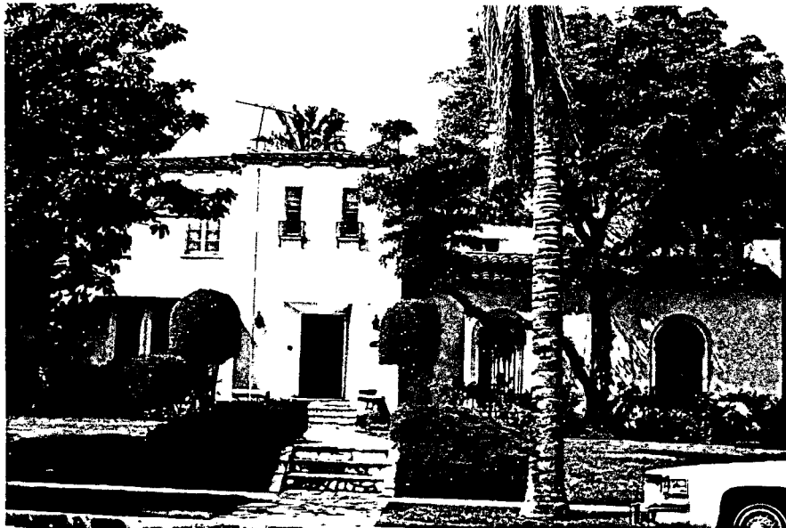
3839 LINDEN AVENUE (1932) - Spanish Colonial Revival 2 story stucco structure with a tile gable roof on right portion and a tile hip roof on 2nd story portion. Wrought iron false balconies over recessed structural opening with flat stepped brick. Semi-circular front windows with more wrought iron. Contractor, L. M. Theleon. (Photo BKL-30)
