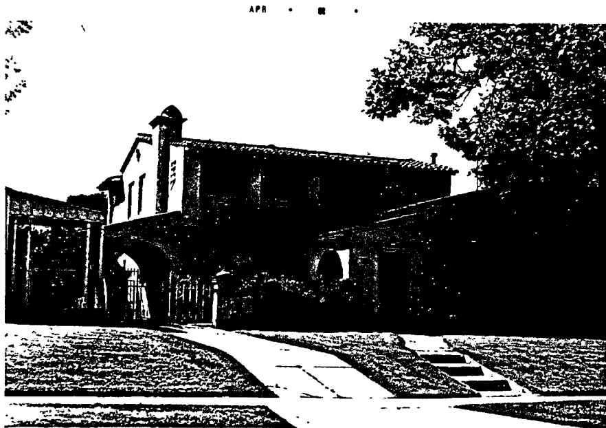
4221 LINDEN AVENUE (1936) - Spanish Colonial Revival two story stucco structure with a tile covered low pitch gable roof. Large open second story balcony. Repeated arch theme on driveway and patio. Wrought iron. Contractor, Russell Mangun Co. (Photo BK2-14)
