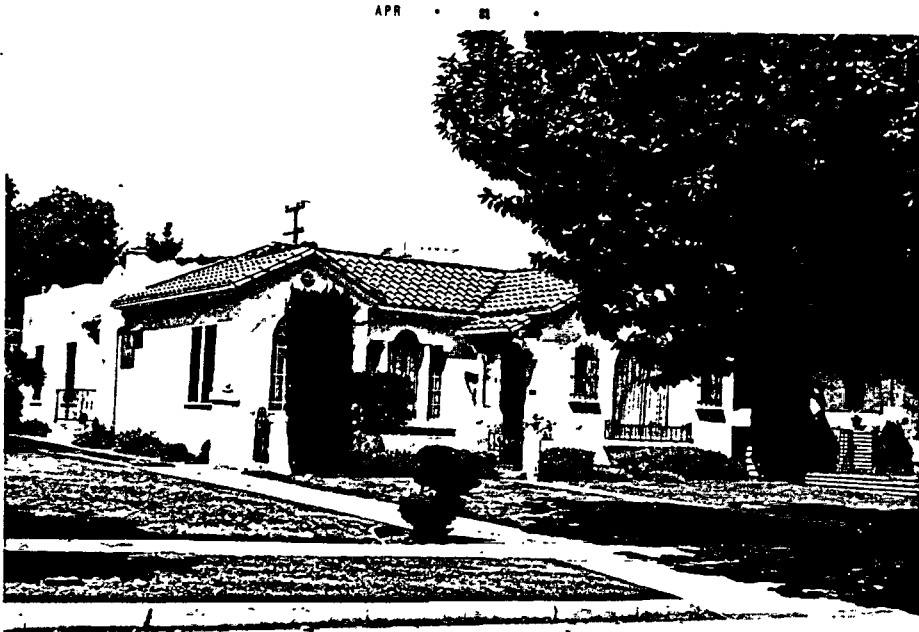
3909 LINDEN AVENUE (1932 - Spanish Colonial Revival stucco cottage with a intersecting tile gable roof in front and a flat roof to the rear with a-mission style parapet. Three sash mission style window with multi-arched side panels, shed porch roof with brackets, and wrought iron in several places along the front. (Photo BKL-33)
