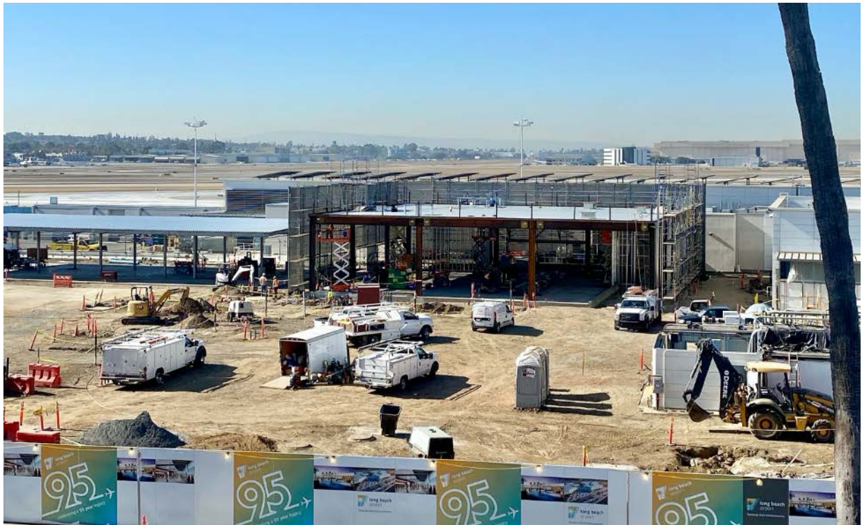
View of CBIS facility with exterior wall framing in place
