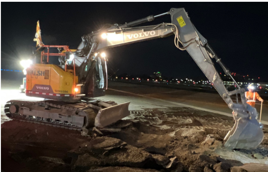
Demolition work in the Phase 4 area
