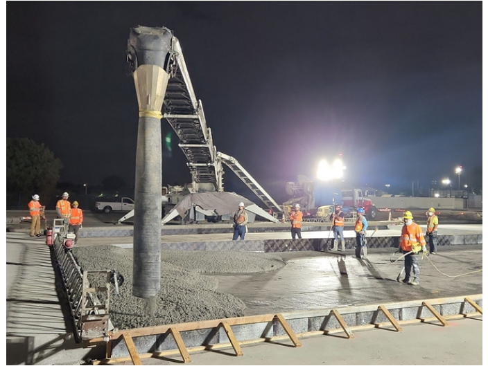
Lean Concrete Base (LCB) placement
