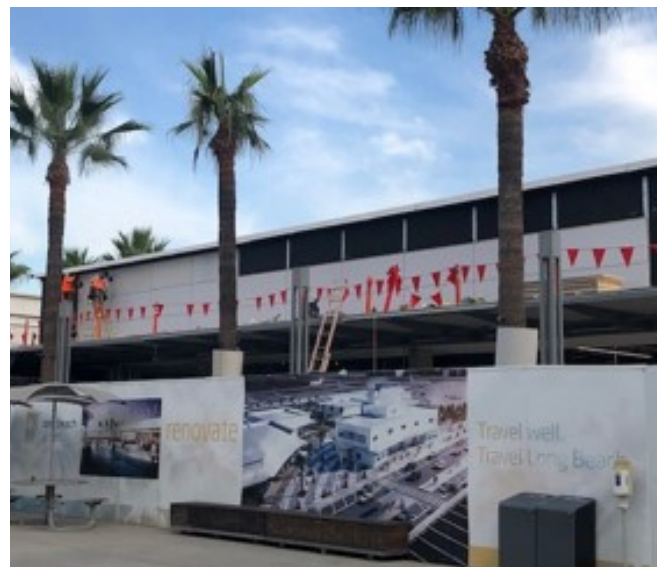
Installation of metal wall panels
