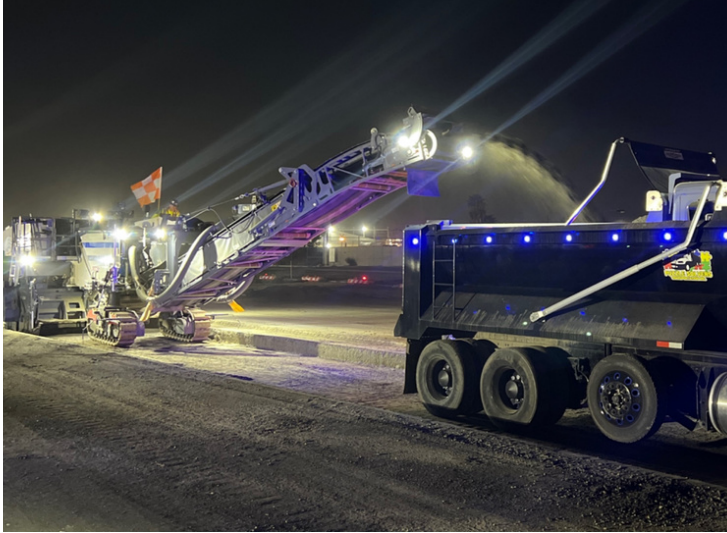
Aggregate base removal in the Phase 3 area
