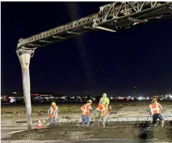
Concrete placement for the Lakewood Tunnel approach
