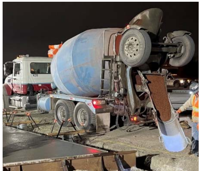
Electrical duct work in the Phase II area
