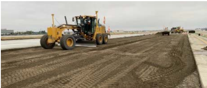
Grading and compaction in the Phase I area
