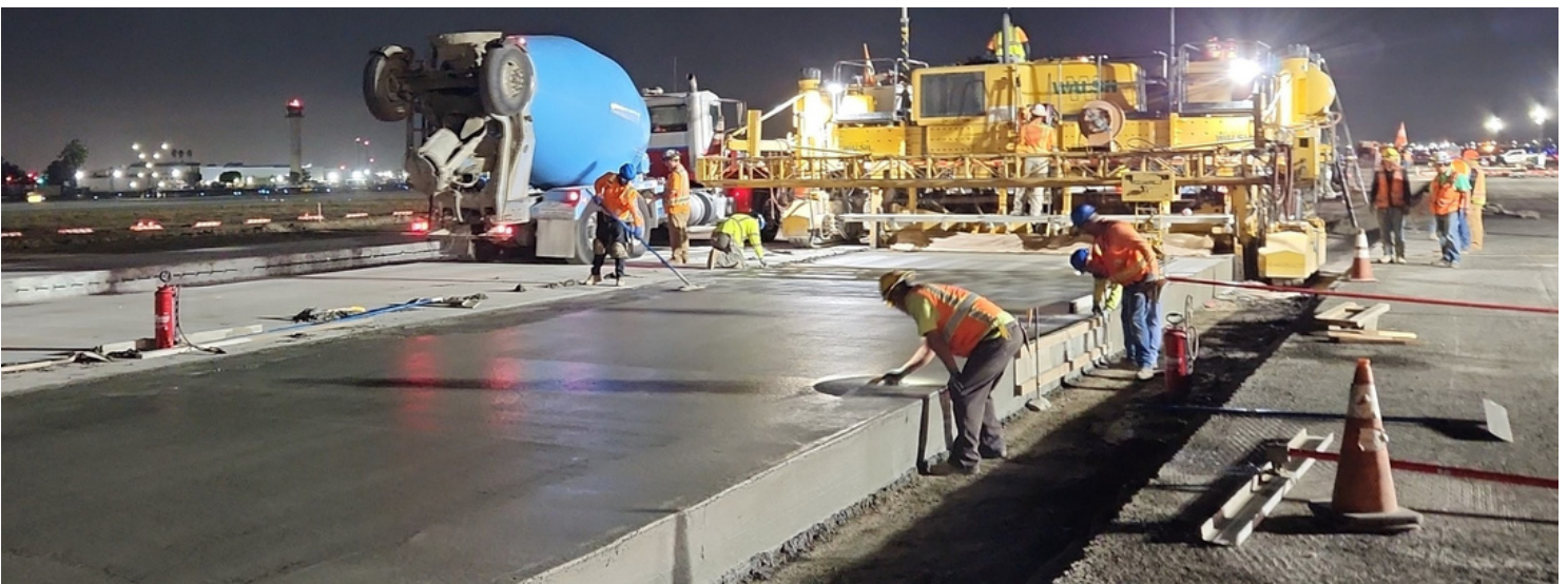
Concrete slipform placement
