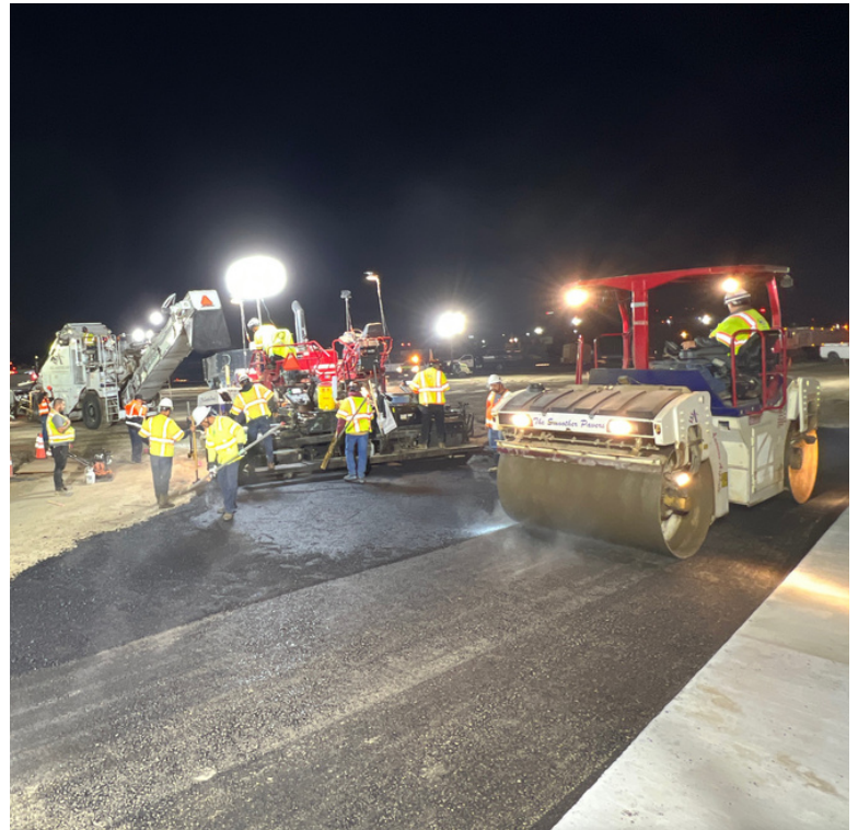
Asphalt pavement placement
