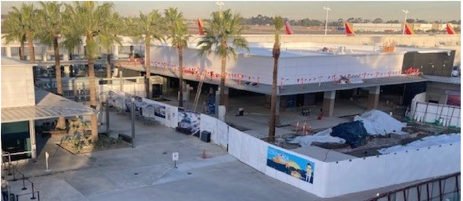
Construction of the New Baggage Claim area continues
