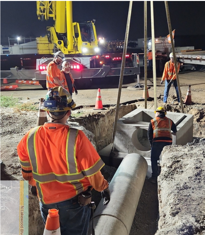
Storm drain installation
