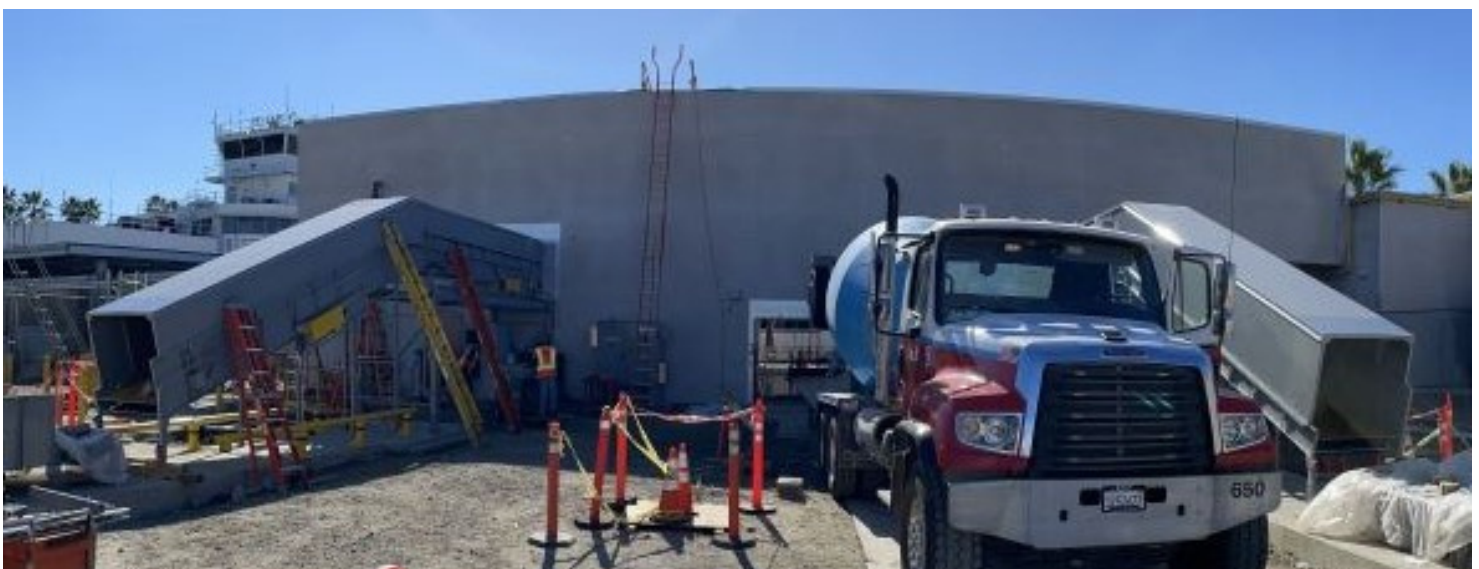
Baggage conveyor installation is underway
