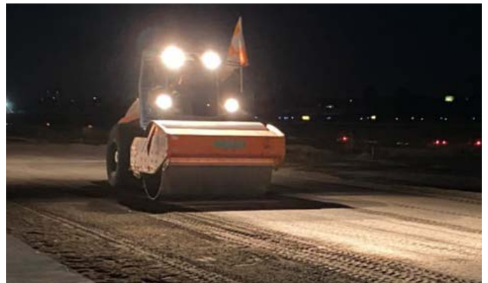
Subbase compaction is underway in Phase V area
