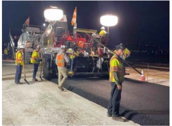
Asphalt paving in Phase I and V areas
