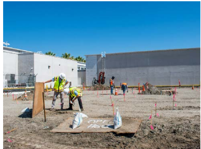
Preparing to install geopiers for the CBIS facility.
