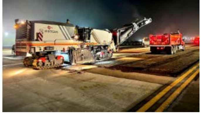
Asphalt milling
