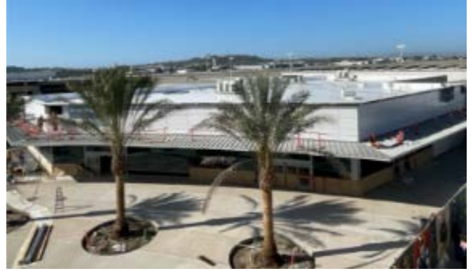
Architectural concrete placement was installed
