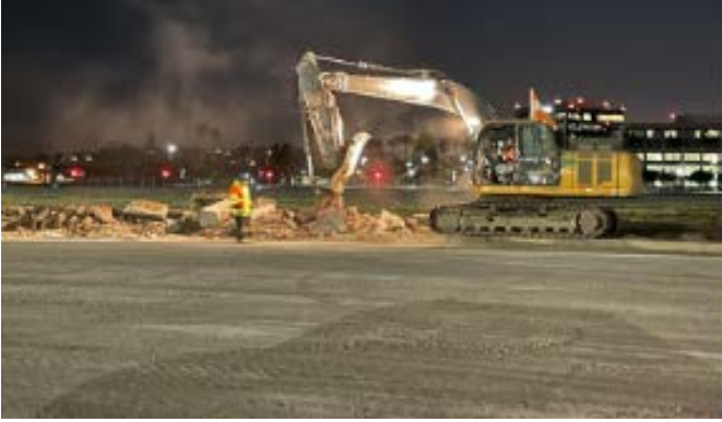
Existing electrical demolition
