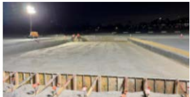
Slab form work
