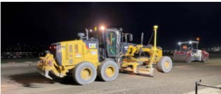
Cement Treated Base (CTB) operation
