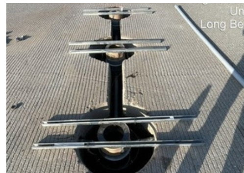
In The Runway 12-30 touchdown zone, barrettes (which each consist of three base cans - represented as three circles) are being removed and replaced
