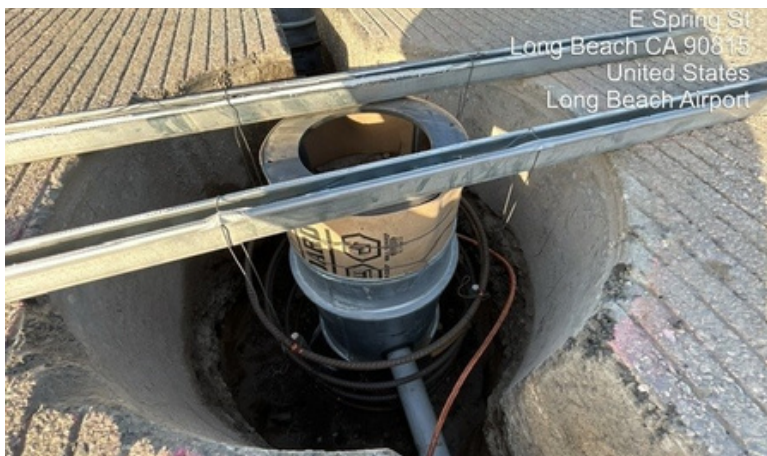
Approximately 180 total base cans, fixtures and transformers will be replaced
