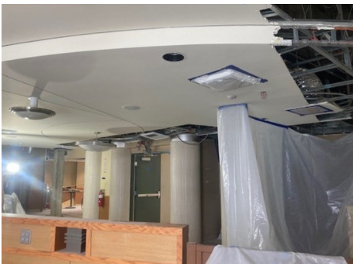
Seismic upgrade work continues in the former 2nd floor event space
