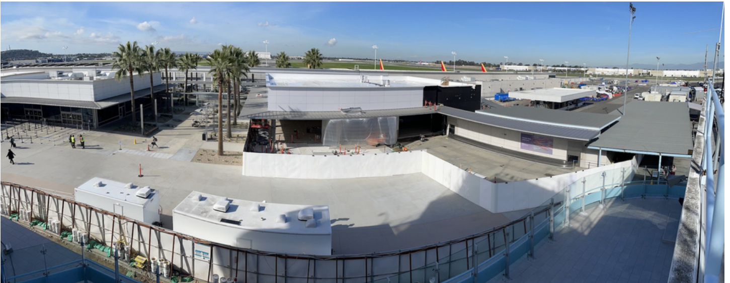
New barricade layout around Baggage Claim #1 and temporary restroom trailers
