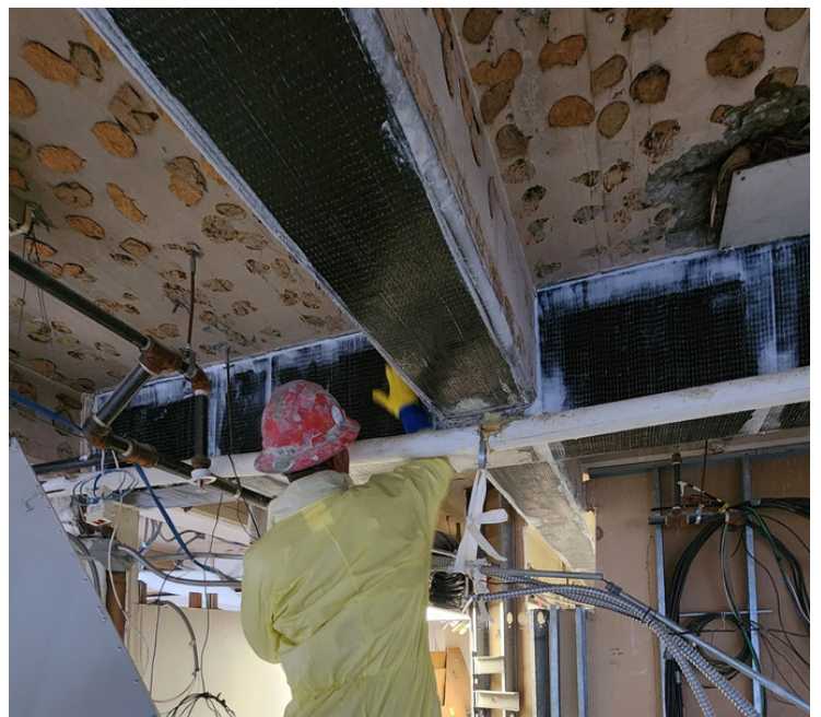
Fiber Reinforced Polymer work was completed in the Historic Terminal
