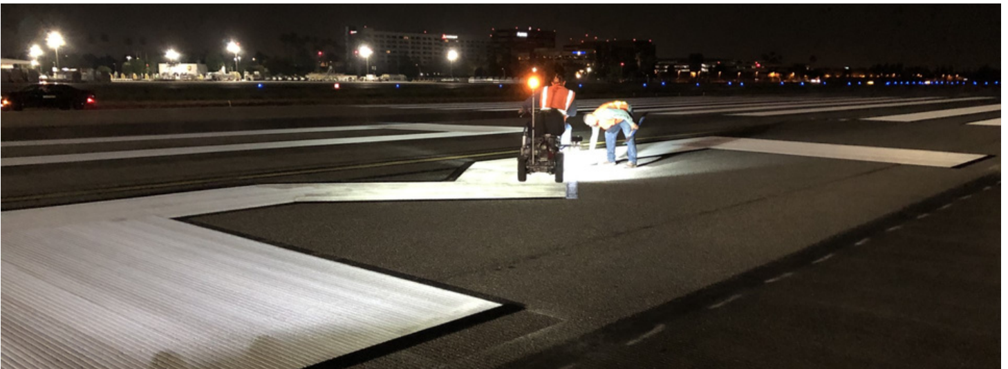
Refreshing airfield striping of runway markings
