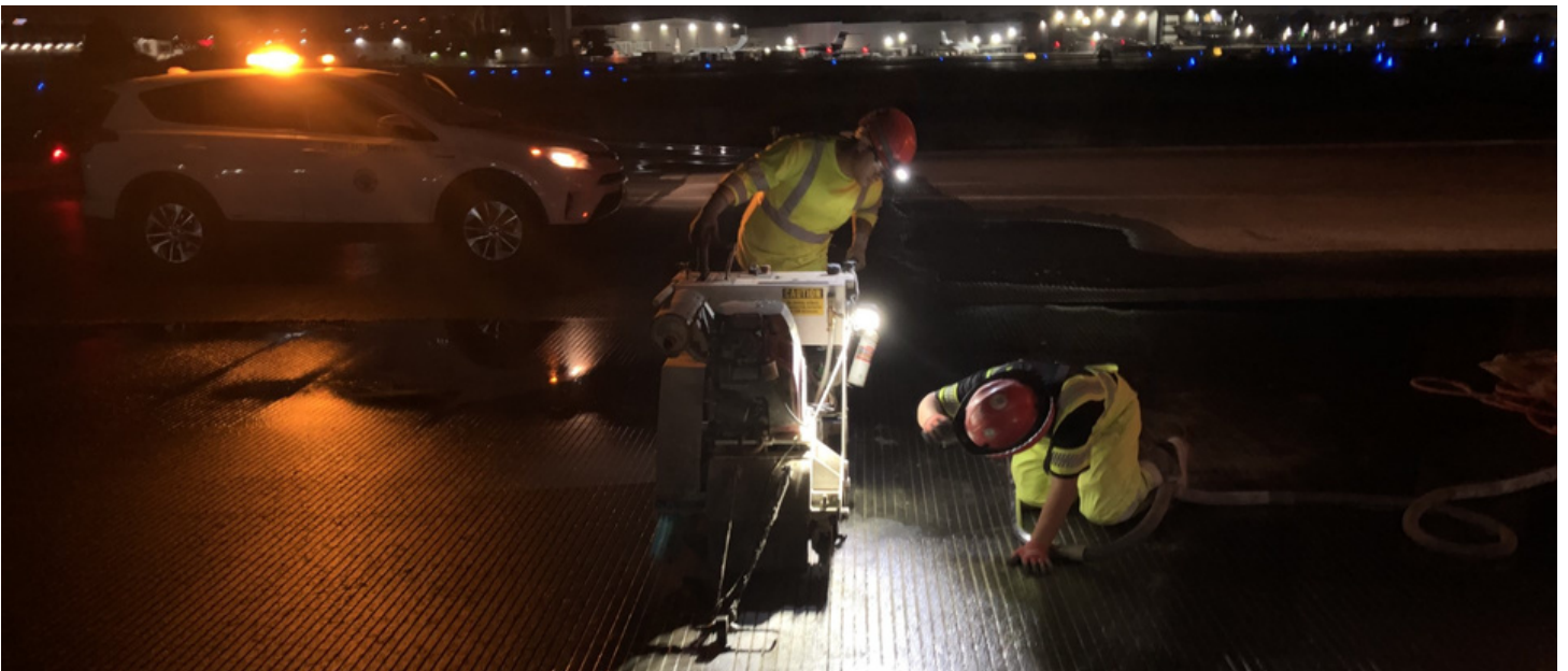
Grooving of airfield pavement
