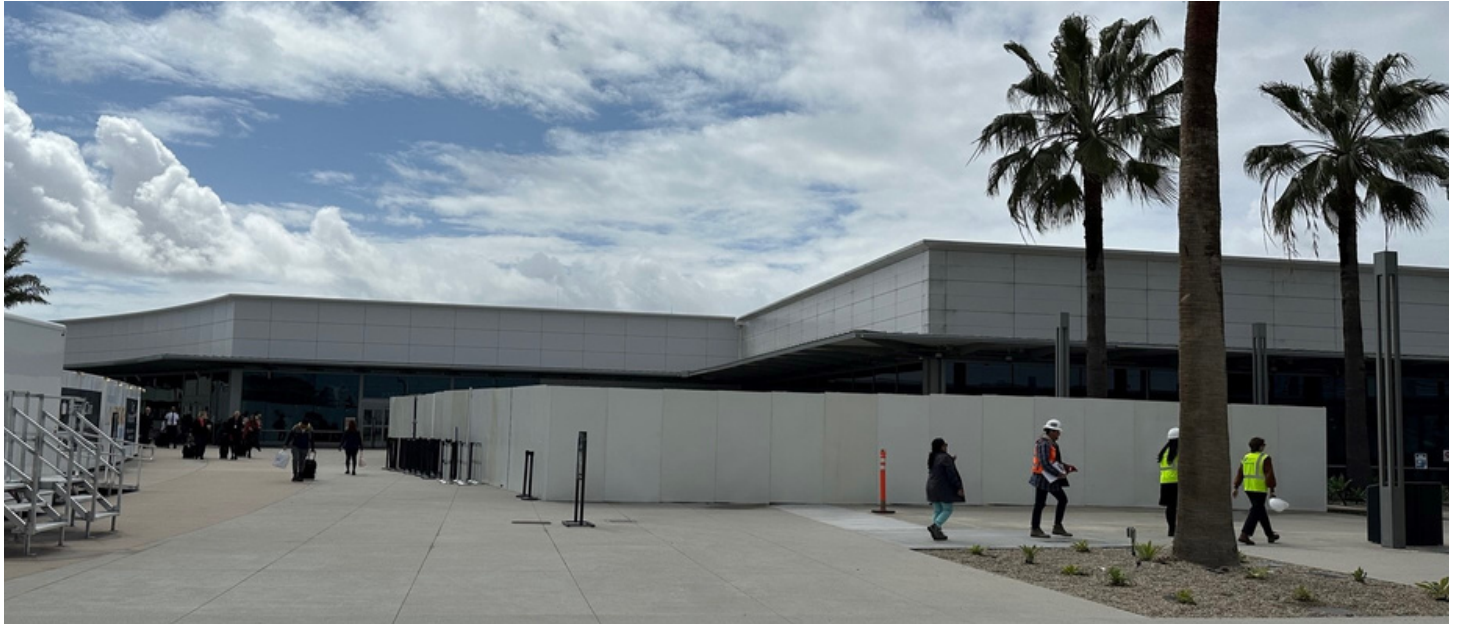
A new canopy for the security screening queue is under construction
