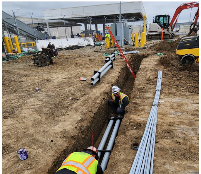
Excavating and underground electrical work for the new BSO and concession is underway
