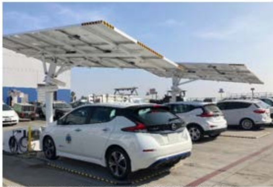
Solar Powered Level II EV Chargers at Fleet.
