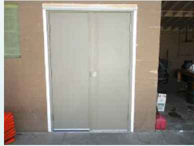
Facility Maintenance staff members Sabino Rodriguez, Luis Oviedo, Pedro Sosa and Dave Hackett replaced doors at Scherer Park.
